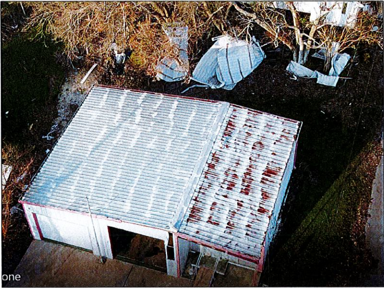
AERIAL VIEW OF DAMAGED SUBROOF WITH DAMAGED PRIMARY ROOF IN BACKYARD
